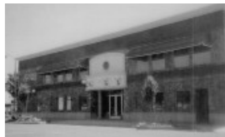
City Hall returns to Turlock's downtown by renovating an early 1900s building.
