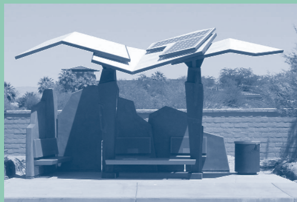
PVs provide the energy for lighting at this Palm Desert bus shelter
